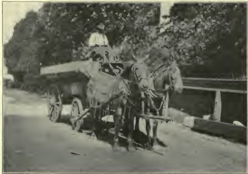
FIG. 35. BARE GROUND AREAS. The view shows a team road, September 4, 1914. Bare ground when subjected to team traffic readily pulverizes to a fine dust which is easily borne on the air currents.
